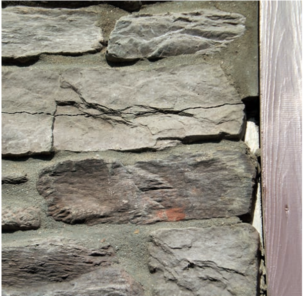
In the pictures Installation on ventilated wall you can note the split created by the strong tensions due to a wrong substructure made of wooden posts to which cement sheets were fixed.
