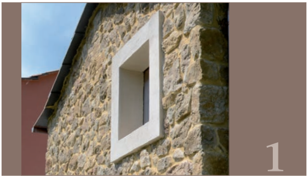
Window edge with frame finished and coloured
