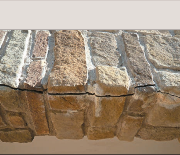
The photograph shows the crack caused by a lack of waterproofing on the wood base. The penetrating water, or even just the dampness, has caused the materials to expand and their movement has split the stone at the corners.
