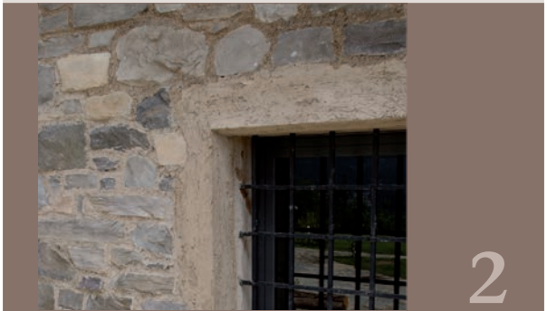
Window border with stones embedded flush
