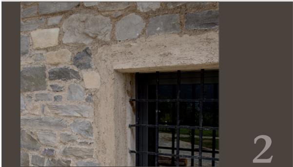
Window border with stones embedded flush
