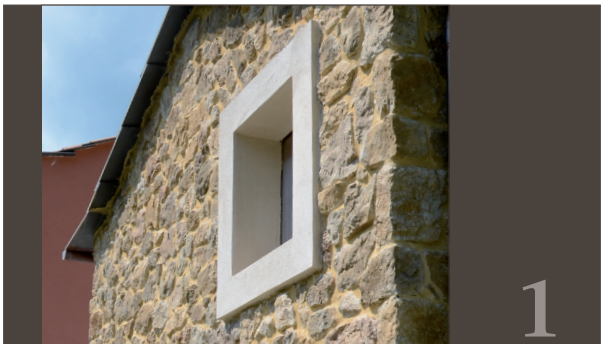
Window edge with frame finished and coloured
