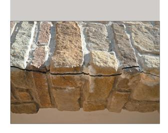
**The photograph** shows the crack caused by a lack of waterproofing on the wood base. The penetrating water, or even just the dampness, has caused the materials to expand and their movement has split the stone at the corners.
