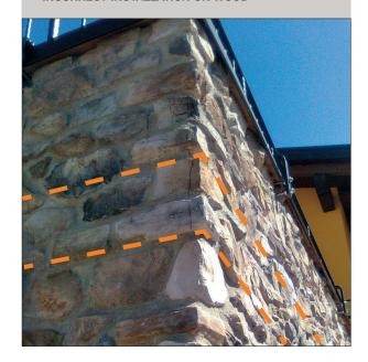
The photograph shows cracks at the corners at the level of the loadbearing slab, where an OSB panel was screwed **directly onto the horizontal laminated beam**. The beam expanded and triggered sufficient forces to break the end section of the glued stone.
